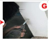
Remove the Frame & Drill the marked positions on the wall.
