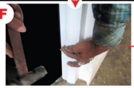
Mark on wall the Drilled position for Roll plugs.
